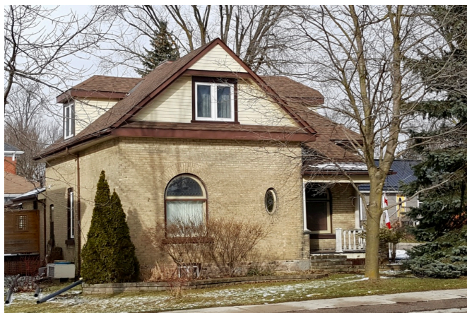
Lot 21, Concession 6, South Easthope Township Plan 307 - Lot No. 62 on the North Side of Hope Street West of William Street
