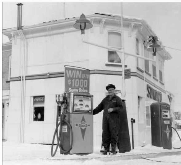
Schaefer's Sunoco Station, 5 Woodstock Street North
