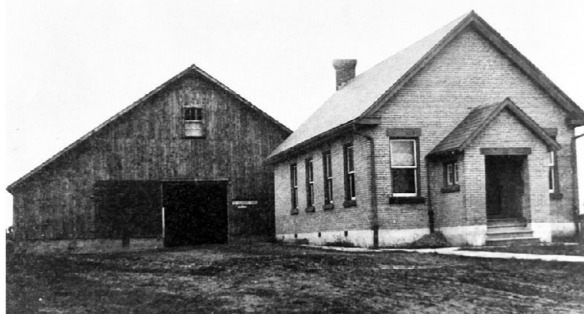
Shed and Township Office built 1905
